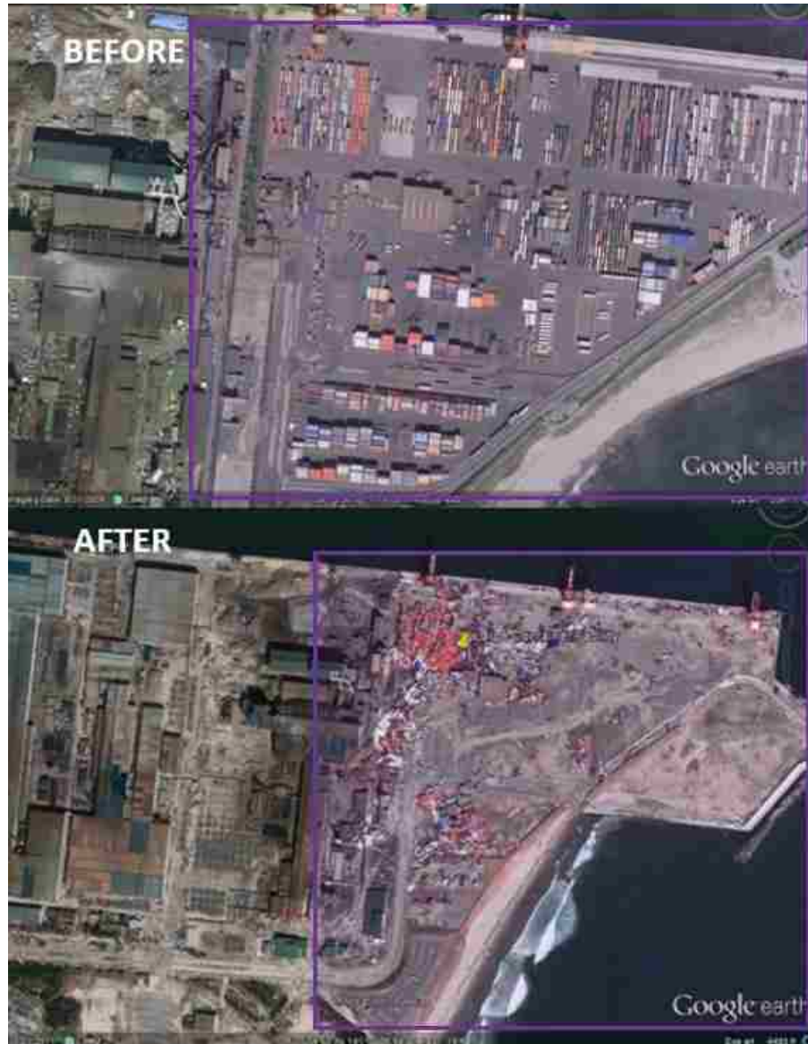
Figure 4: Sendai large container facility before and after
